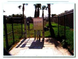
A LS is a facility for elevating the wastewater (sewage) from your property or business and transporting it to a private or municipal treatment system. LS's consist of a below-grade wet well, pumps and floats, discharge piping, and an above ground control panel housing the electrical components, pump switches, and highlevel emergency alarms.
